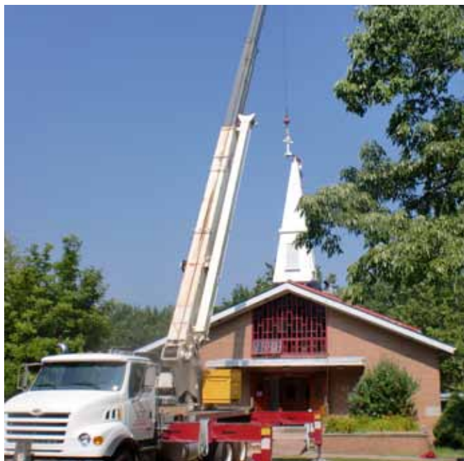
A cell tower in disguise gave St. Gregory's back its steeple and a thumbs up from its neighbors.
